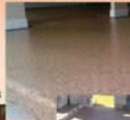
Garage floor Epoxy Chip Flake
