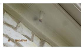
The tube coming out of the soffit is the secondary drain for your AC condensation. The secondary drains on homes with the condenser in the attic always have the secondary drain outlet positioned over a window so that the homeowner will notice it dripping.
